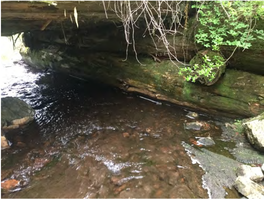
Right Bank Abutment when facing downstream
