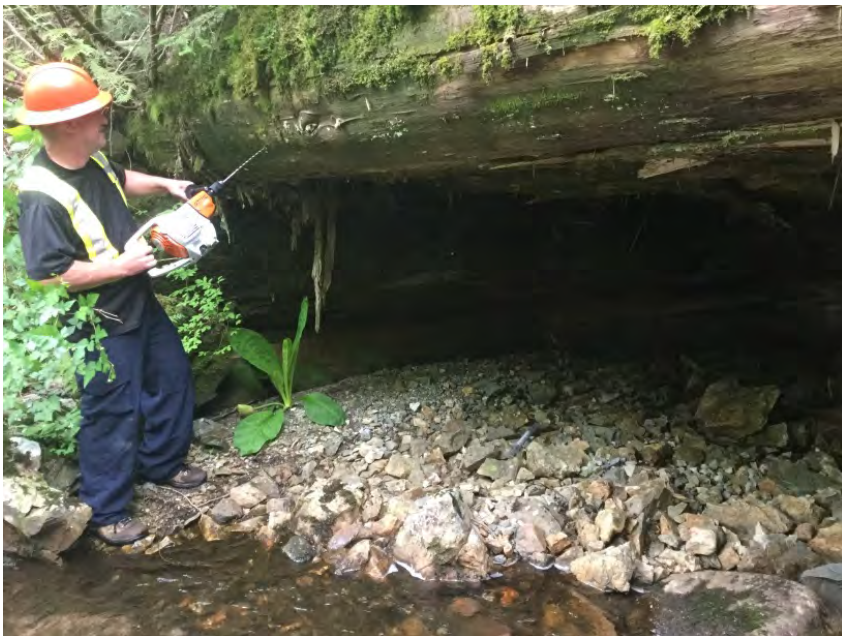
Left Bank Abutment when facing downstream
